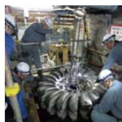
Replacement of hydraulic turbine runner
