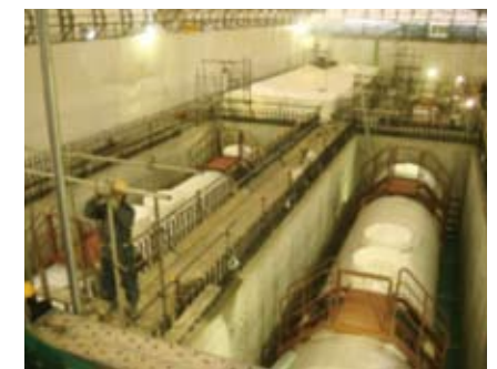
Installation of underground gas oil storage tank
