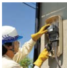
Scene of smart meter installation
