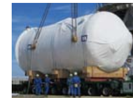
Installation of filtered vent equipment for containment vessel
