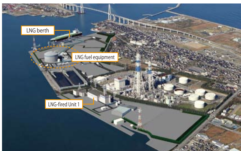
Conceptional image of LNG-fired Unit 1 of Toyama Shinko Thermal Power Station
