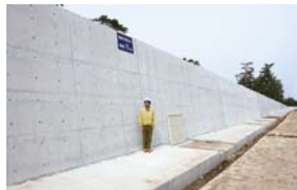
Installation of tide embankment
