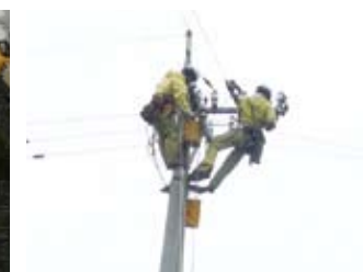
Recovery work on the pole
