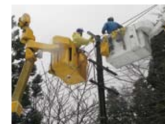
Recovery work at mountainous area
