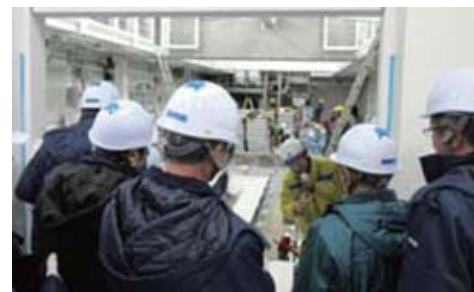
Scene of site visit (construction of expanded emergency measures facility)
