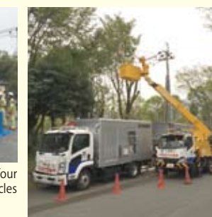
Work to connect high voltage power generation vehicle with power line
