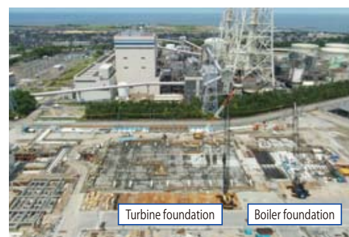
Construction of LNG-fired power generation equipment
