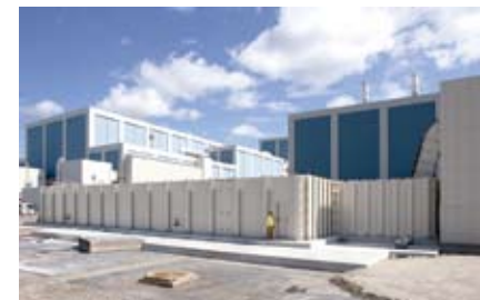
Installation of tide barrier
