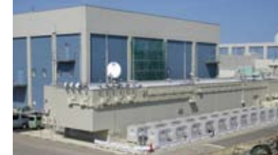
Appearance of expanded command & control area (expanded emergency measures facility)
