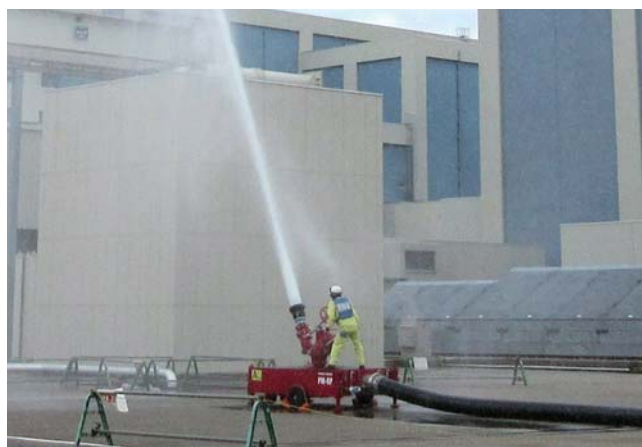
Training in the Operation of the Water Sprayer
