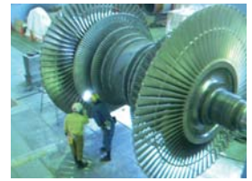
Regular inspection of a thermal power station
