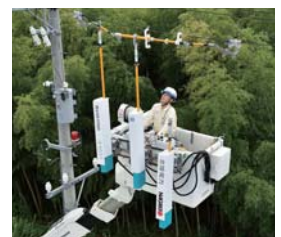
Power cable cutting and connection work
