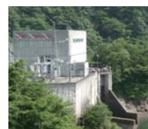
Arimine No. 2 Power Station
